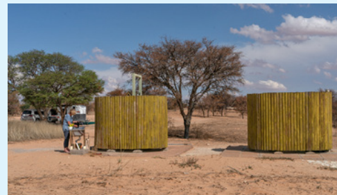
Image of enclosures of long drop toilet on right and cold water bush shower on left (Botswana)
